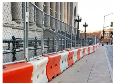
Water-Wall Fence attached for additional job-site security.
